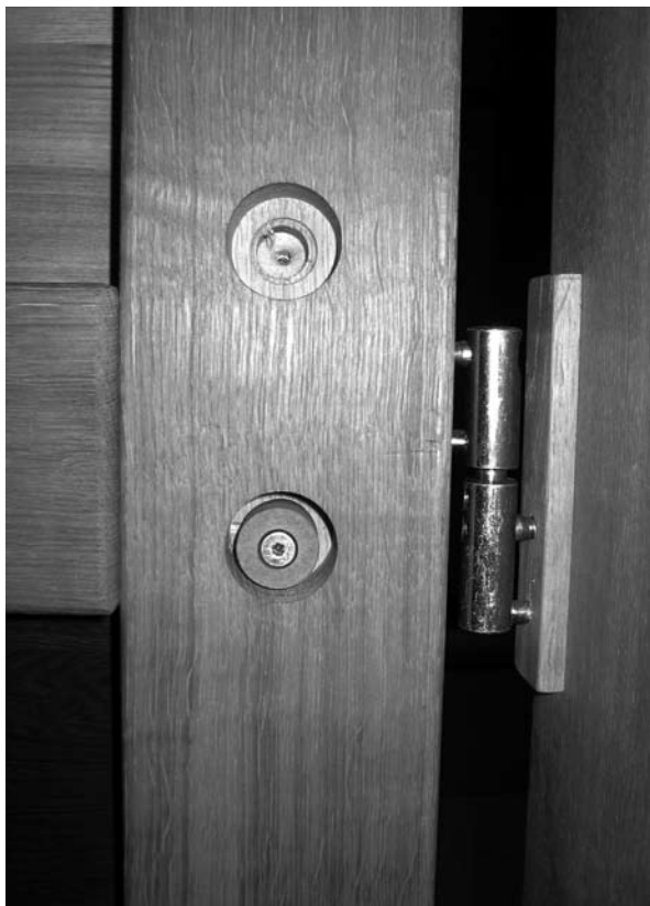
Figure 2. Detail view of the first Door bolt assembly, one bolt removed.
