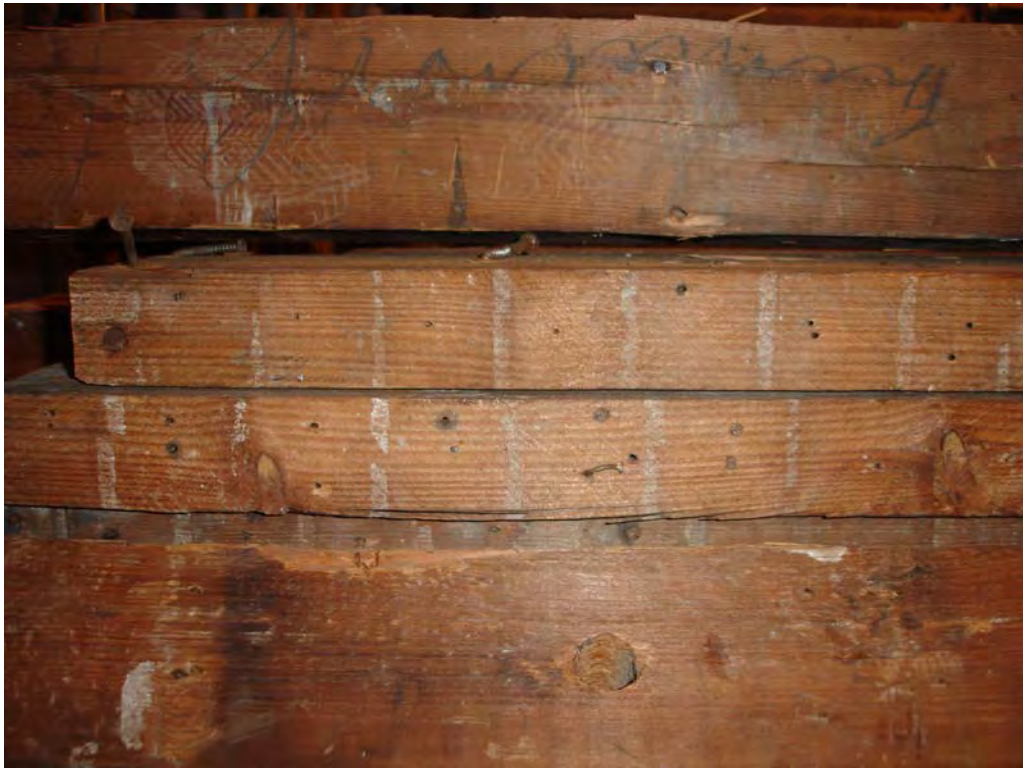
The raw material, showing plaster lath marks. In several places there is writing in pencil in a florid script which likely is of the original builder. Many nails and tacks had to be removed.
